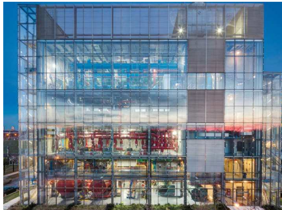
University of Chicago West Campus Combined Utility Plant
