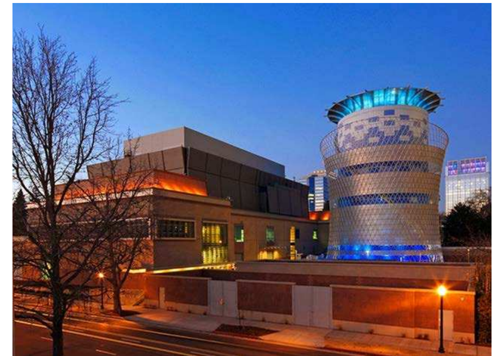
California Dept. of General Services Central Utility
